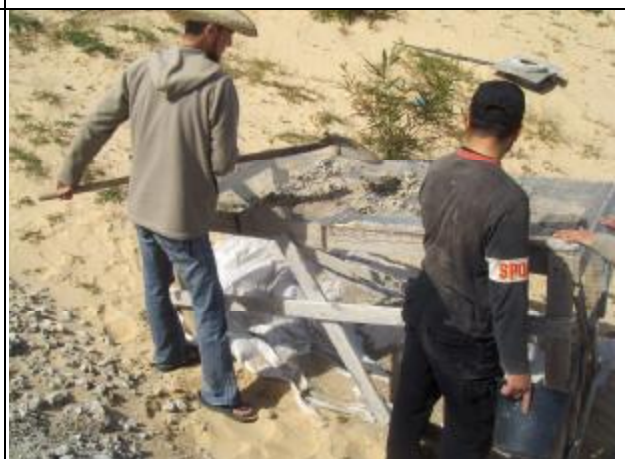
Figure B6:Sieving recycled aggregate
